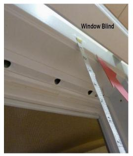
Photo shows a close up of the top of the window. Guard is mounted inside, close to window; blind is installed on the outside casing.
